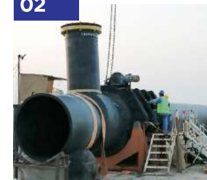
Desalination Plant Intake and Outfall Pipeline-RAK
