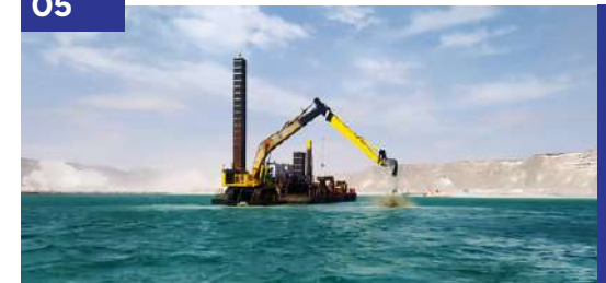
Seawater Intake and Outfall for Crude Oil Park-Oman
