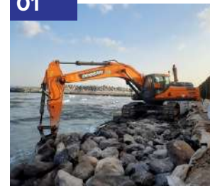
Collecting and Extending of TSE Outfall to Sea-Sharjah
