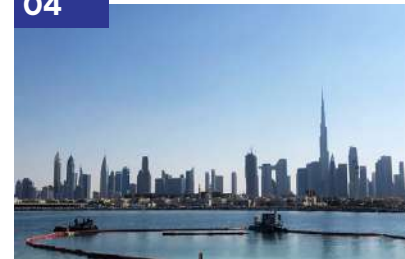
Stormwater Outfall Lines-Dubai
