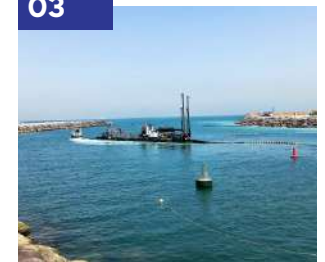
Channel Dredging - Sharjah
